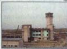
The air traffic control tower is 97% complete
